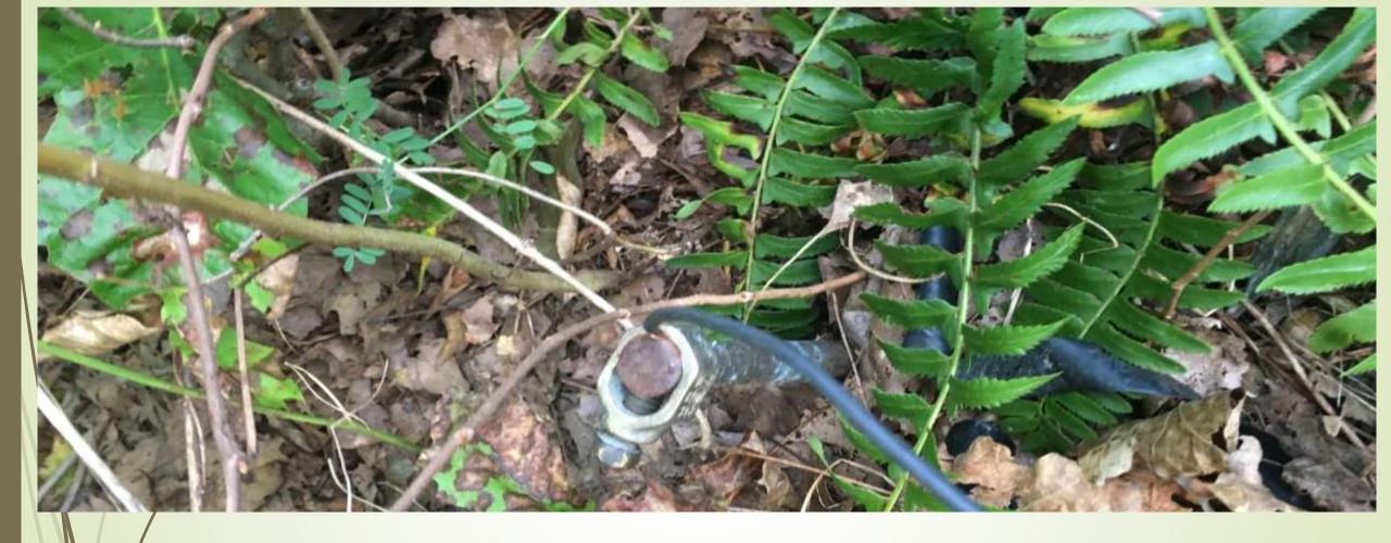
Antenna grounding rod w/10awg wire to antenna wires
